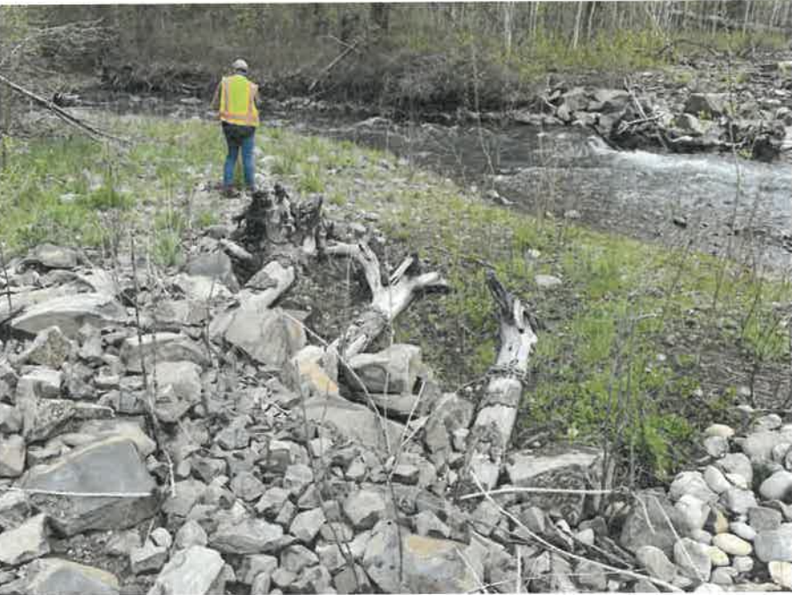
PHOTO 11: Engineered bank armoring 3 miles upstream of Site
